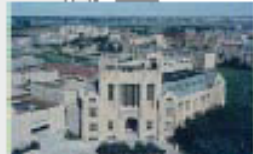
⑪ THORVALDSON PROJECT, CHEMISTRY, SSSC & COMPUTER SCIENCE RENOVATIONS 1924 & 1966 WING | 2004
