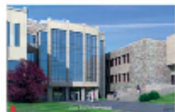
13 PLACE RIEL EXPANSION/ RENOVATIONS |2011 $28.35M
