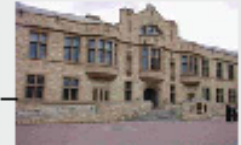
⑨ COLLEGE BUILDING RESTORATION/RENOVATION | 2003 $20.25M
